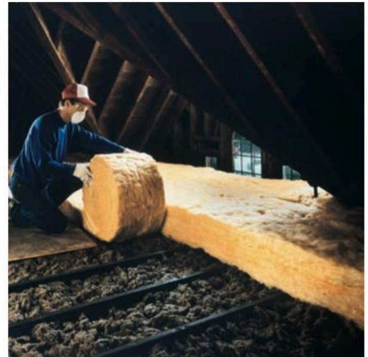
Layer fiberglass roll insulation perpendicular to the joists.
